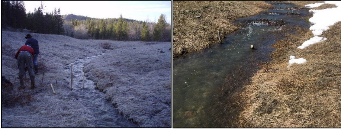
Figure B-28. California Creek pre- (2015) and post-restoration (2017) photos.
